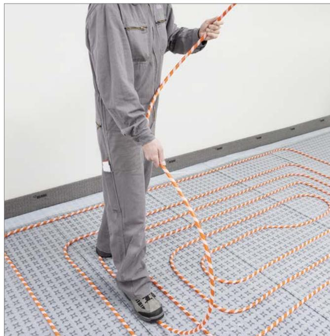
Abb. 2-6 RAUTHERM SPEED plus Rohrinstallation
