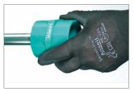
2 Carefully deburr the pipe ends, internally and externally, using a suitable deburring tool (e.g. pipe deburring tool). Carefully remove any saw filings and deburring residues. The pipe end should be clean, have no sharp edges, with a resulting small smooth chamfer applied as a result of the deburring process. Clean pipe ends with suitable abrasive wool pad.
