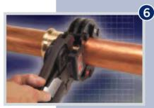
On completion of the pressing operation an audible bleep will be heard; disengage the adaptor by depressing the jaw levers and remove the collar from the fitting. See below for 108mm fitting.
