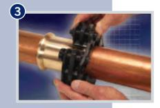
Ensure that the groove in the collar corresponds to the bead on the fitting and that the support plate on the collar fits over the tube side of the joint.
