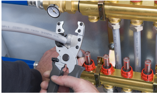
Fig. 1: Before connecting the heating circuit to manifold cleanly cut off FH composite pipe in the correct length.
