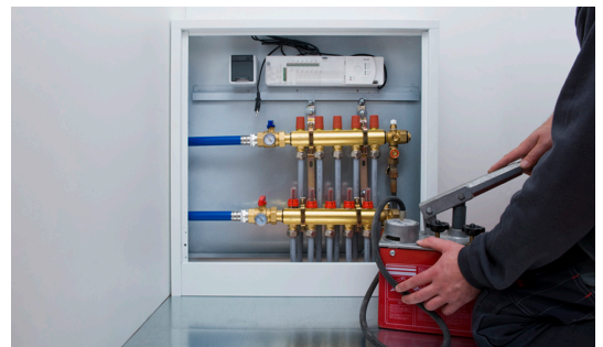
Fig. 6: Label the individual heating circuits. Carry out pressure test in accordance with the pressure test protocol.
