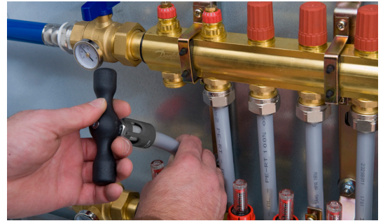
Fig. 2: Centre pipe and bevel with beveling tool - 2 mm all round bevel on inner pipe.
